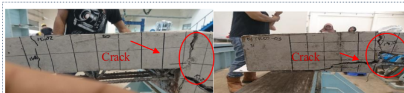
Figure 2. The crack at support.
